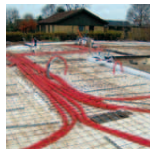
Example of NilAIR installed in the floor (ground cover) of a detached house.
